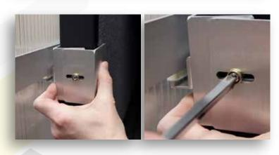
5. ONCE IN PLACE, SECURE THE BRACKET BY SQUEEZING AND TIGHTENING THE SCREW WITH A PHILLIPS SCREWDRIVER.
